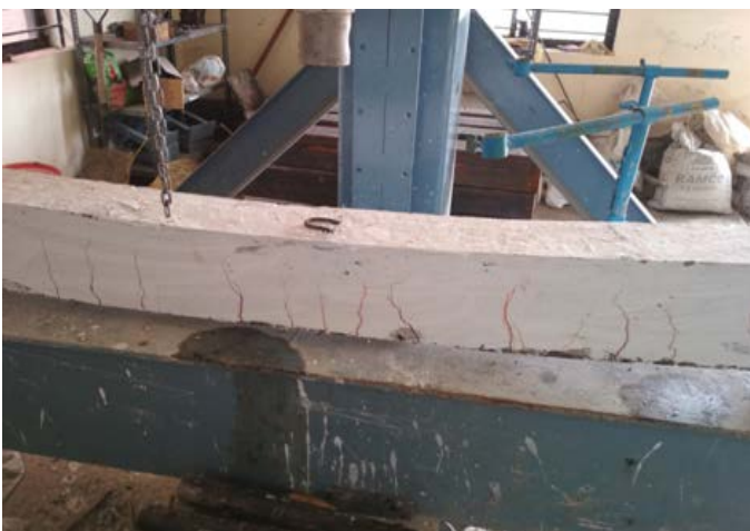
Fig.10 Cracks developed during loading
